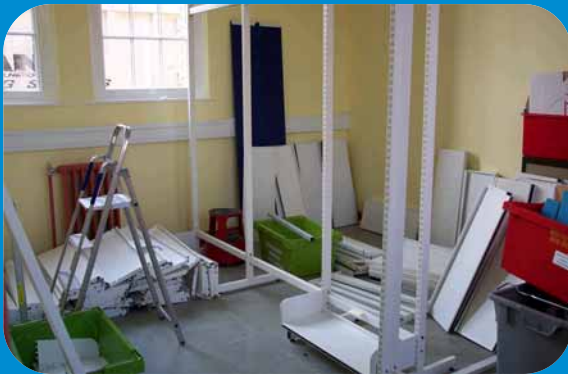
Constructing the library shelving
